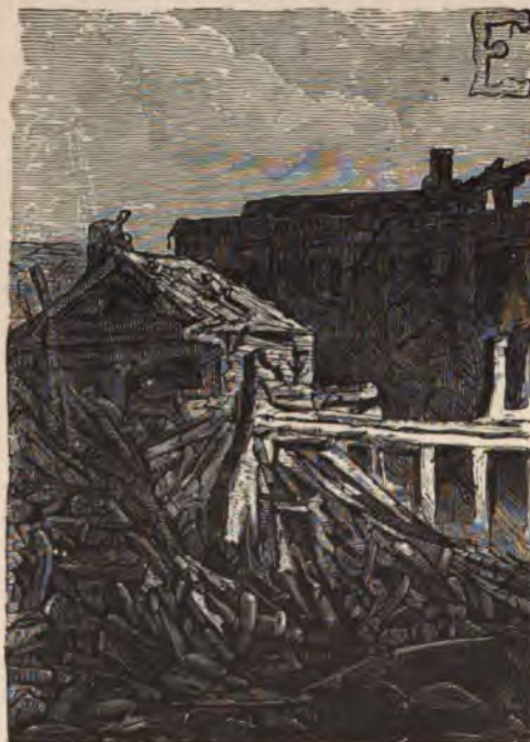
AFTER THE EARTHQUAKE.
